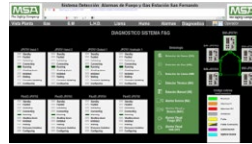
VISTA GENERAL HMI
